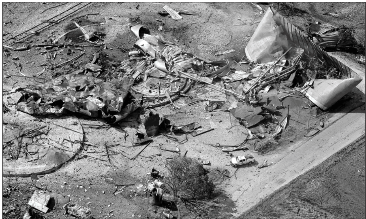
This aerial photograph shows the remains of the West Fertilizer Co. plant that was destroyed by an explosion Wednesday night. A damaged emergency response vehicle is visible in the bottom left. The plant was built in 1960. The town of West 'grew up and around that fertilizer plant,' said Gary Payne of Brazos Feed and Supply. TONY GUTIERREZ / ASSOCIATED PRESS
